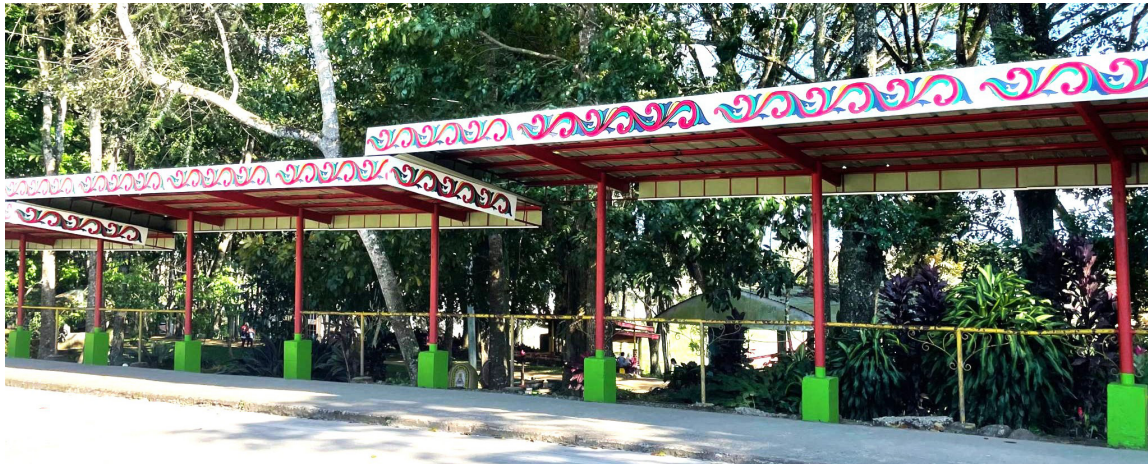
Newly renovated campus covered walkway leading to the Annex Buildings
