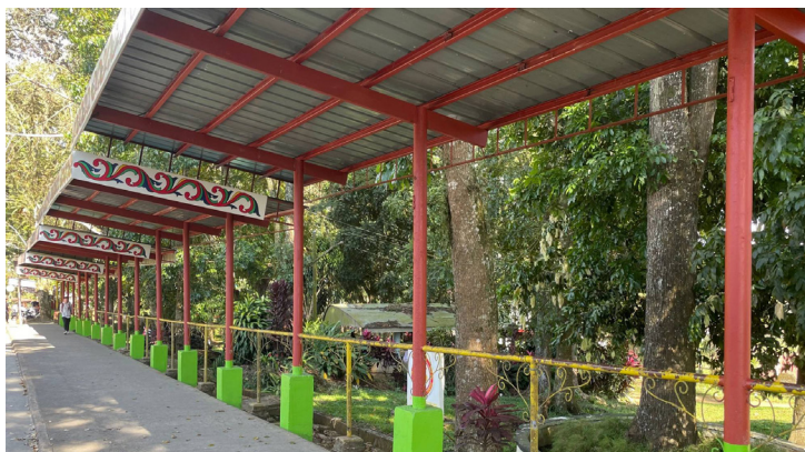
Closer view of the newly renovated campus covered walkway
