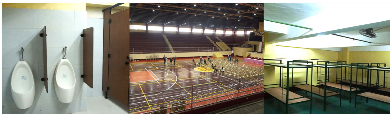
Interior upgrades of the Dimaporo Gymnasium rehabilitation project, showcasing the newly refurbished restroom facilities (left), the fully renovated indoor court and bleachers (middle), and the newly installed hostel accommodations below the stage (right).
